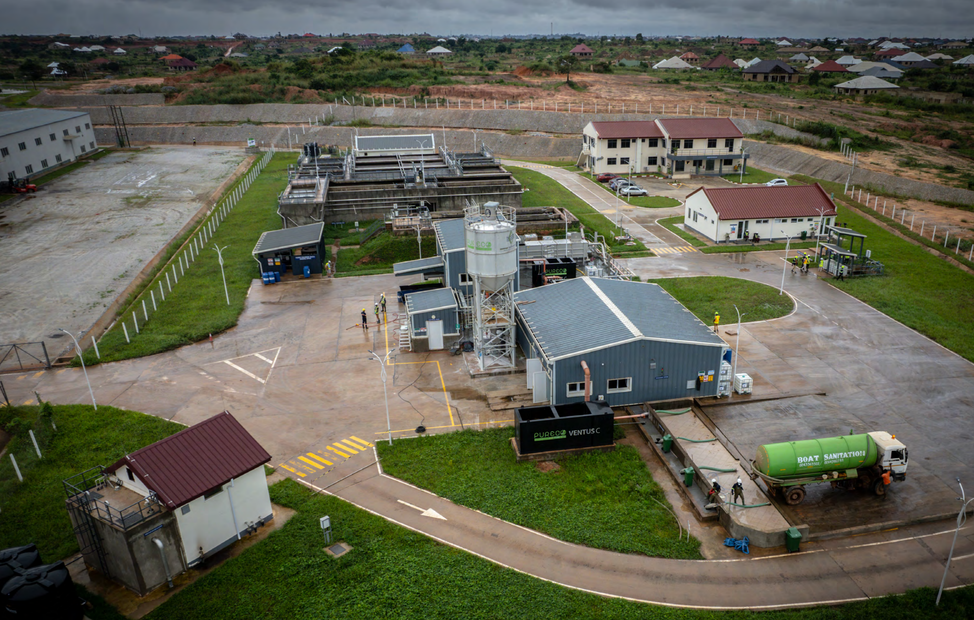
WASTEWATER TREATMENT PLANT, KUMASI, GHANA
